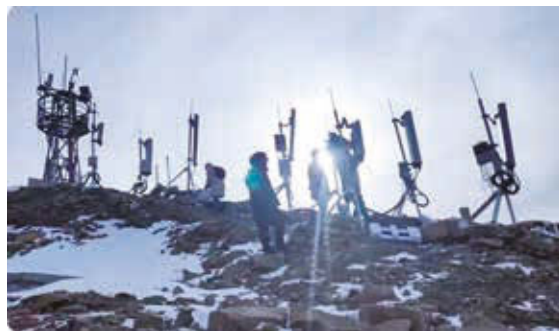
Capinfo employees carefully lay cables and conduct inspections
